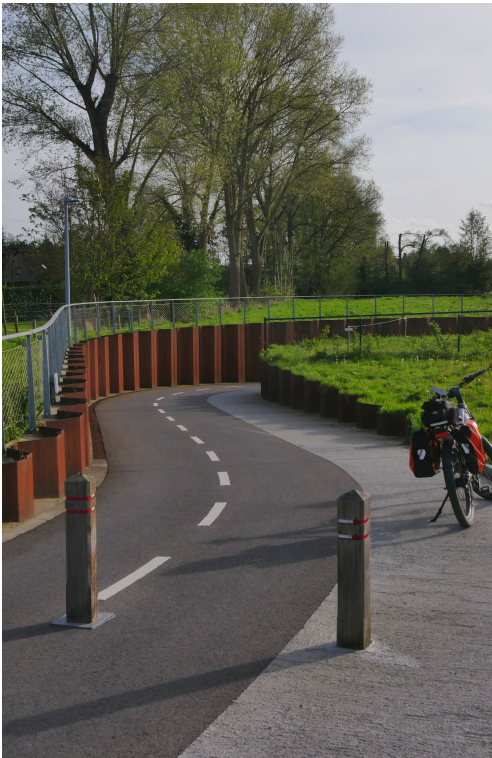
Photo 25 - Cycle and pedestrian tunnel Tonnestraat
