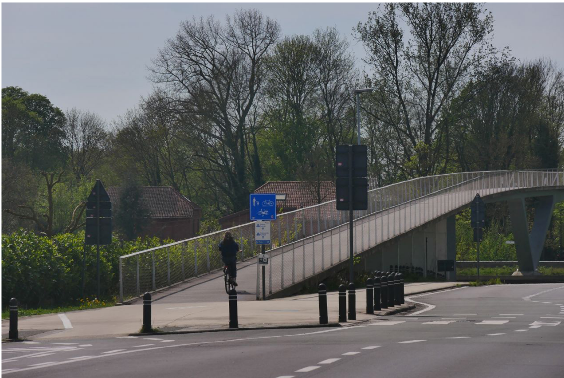
Photo 12 - The start of the ramp of the André Denysbrug.
