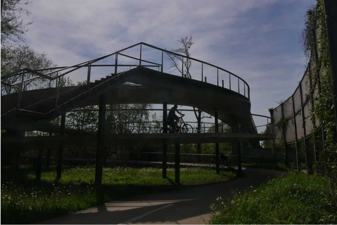
Photo 13 - The spiral ramp
