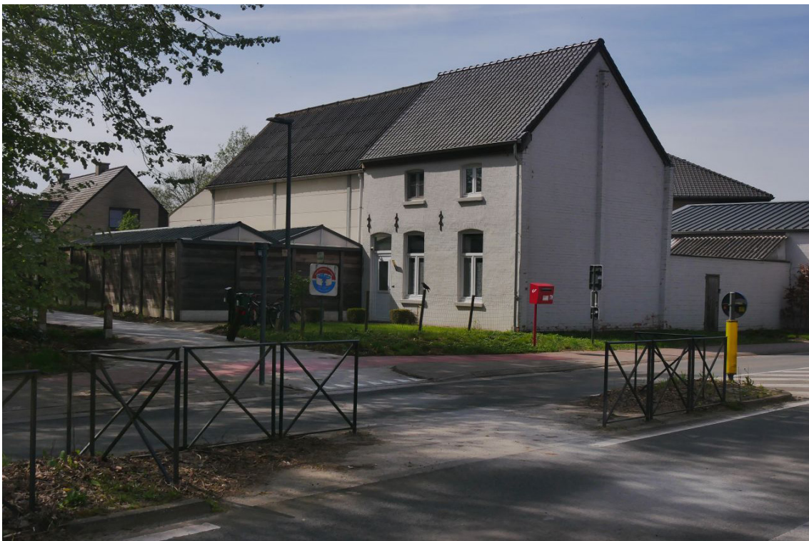
Photo 15 - Crossing construction on Klossestraat
